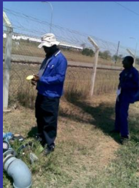
Phase 1 GPS Implementation: meter reading team capturing all existing known connections.
